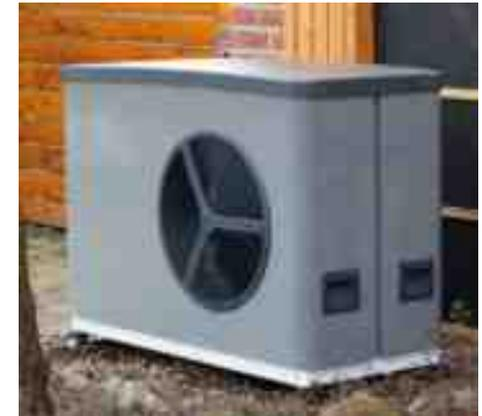
1 kWh Strom = 3 kWh Wärme
